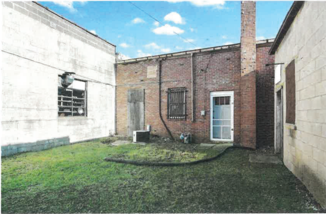
Rear of Building – Visible from Public Alleyway and Park St.
