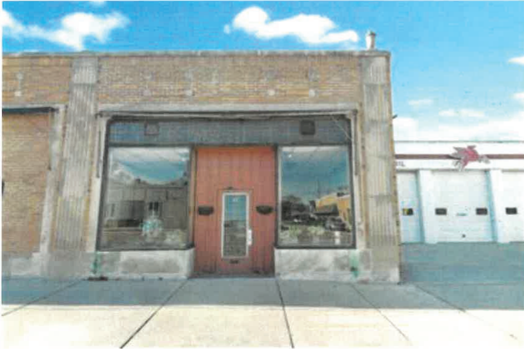
Front of Building – Facing State St. (West Side)
