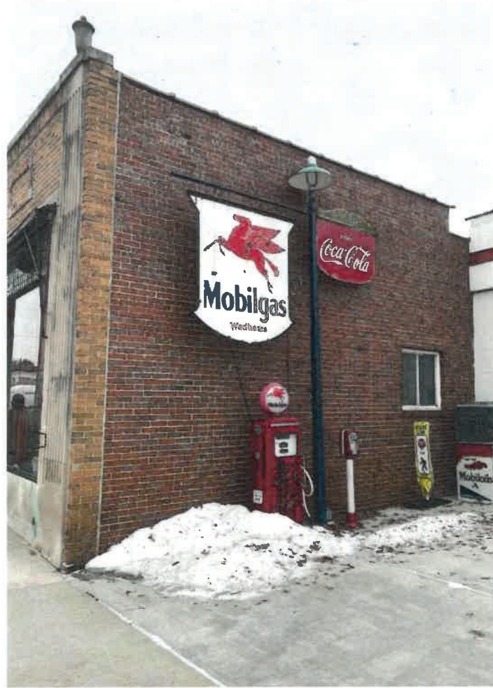
Side of Building – Facing State St. (North Side)
