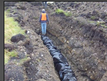
Water Distribution & Storage
