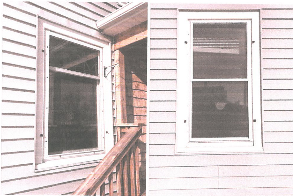
Figure 2: Photo of two different styles of existing windows proposed for replacement
