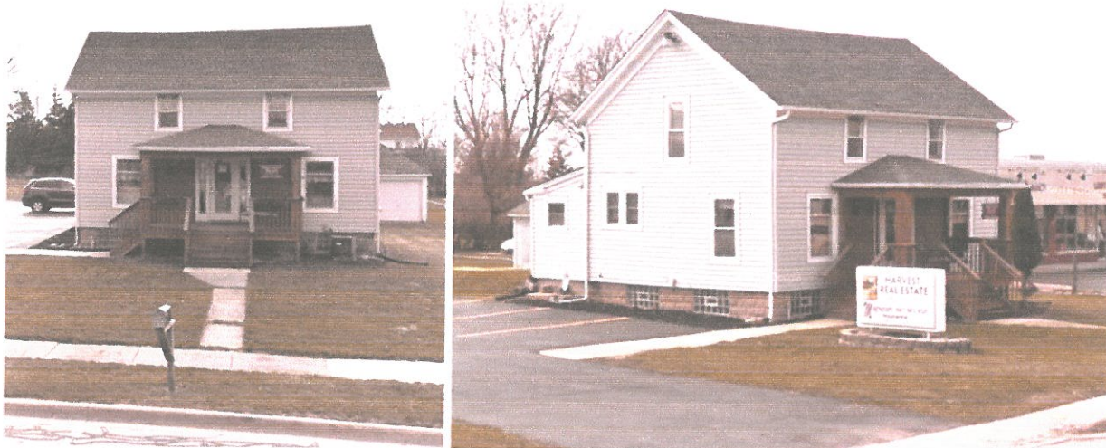
Figure 1: East (left) and South Elevation (right) view of the building from street
