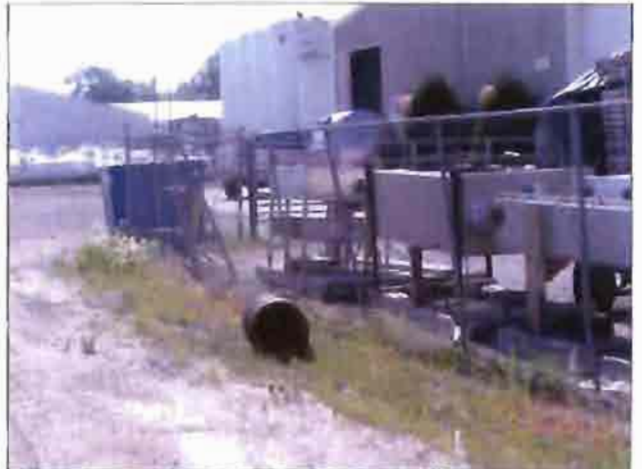
The west side of an Industrial building fronting Mill St. has sections of fence coming down.
